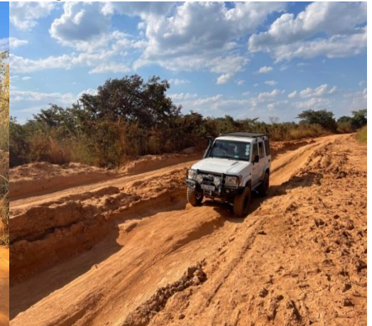
Chainage 86 +000 – Section in poor condition
