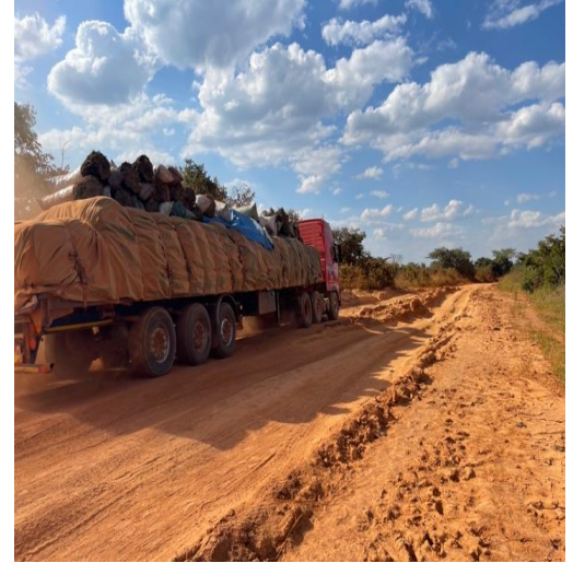
Chainage 86 +000 – HGVs still using the Road
