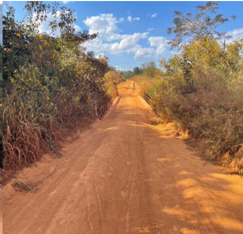
Single lane Mushindamo River Bridge
