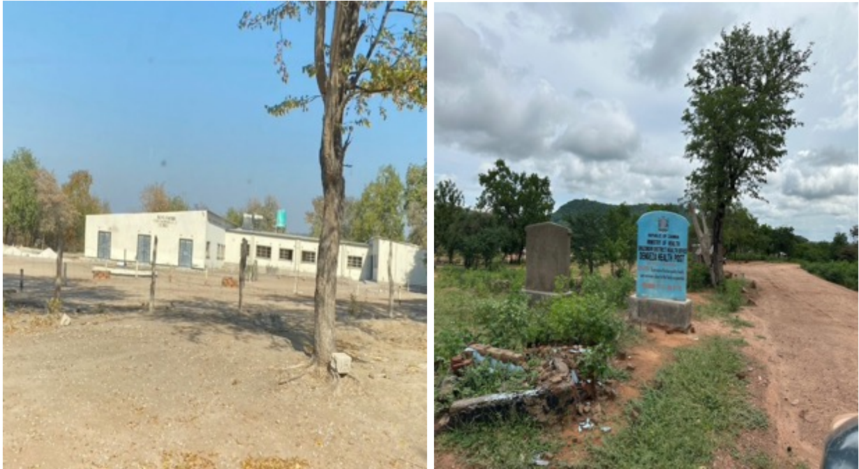
Figure 24: Pictures showing a clinic and health post near the project area
