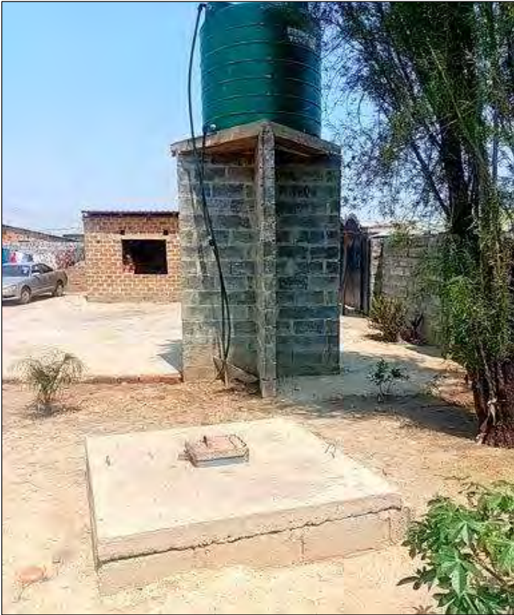
Figure 5-1: Photograph of a protected well in Luangwa Township
