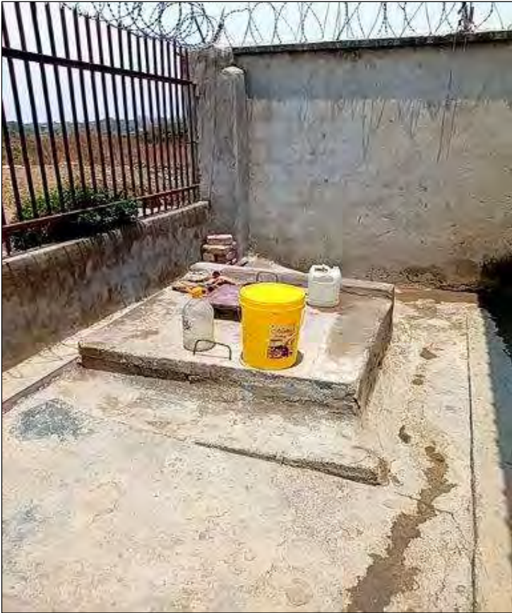
Figure 5-2: Photograph of a protected well in Luangwa Township
