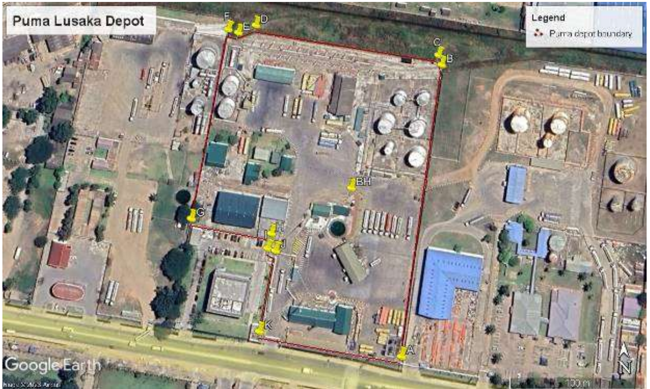
Figure 1: Google Satellite Image of the Site
