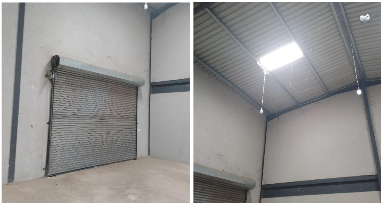
Figure 2: Interior view of the e-waste project facility
