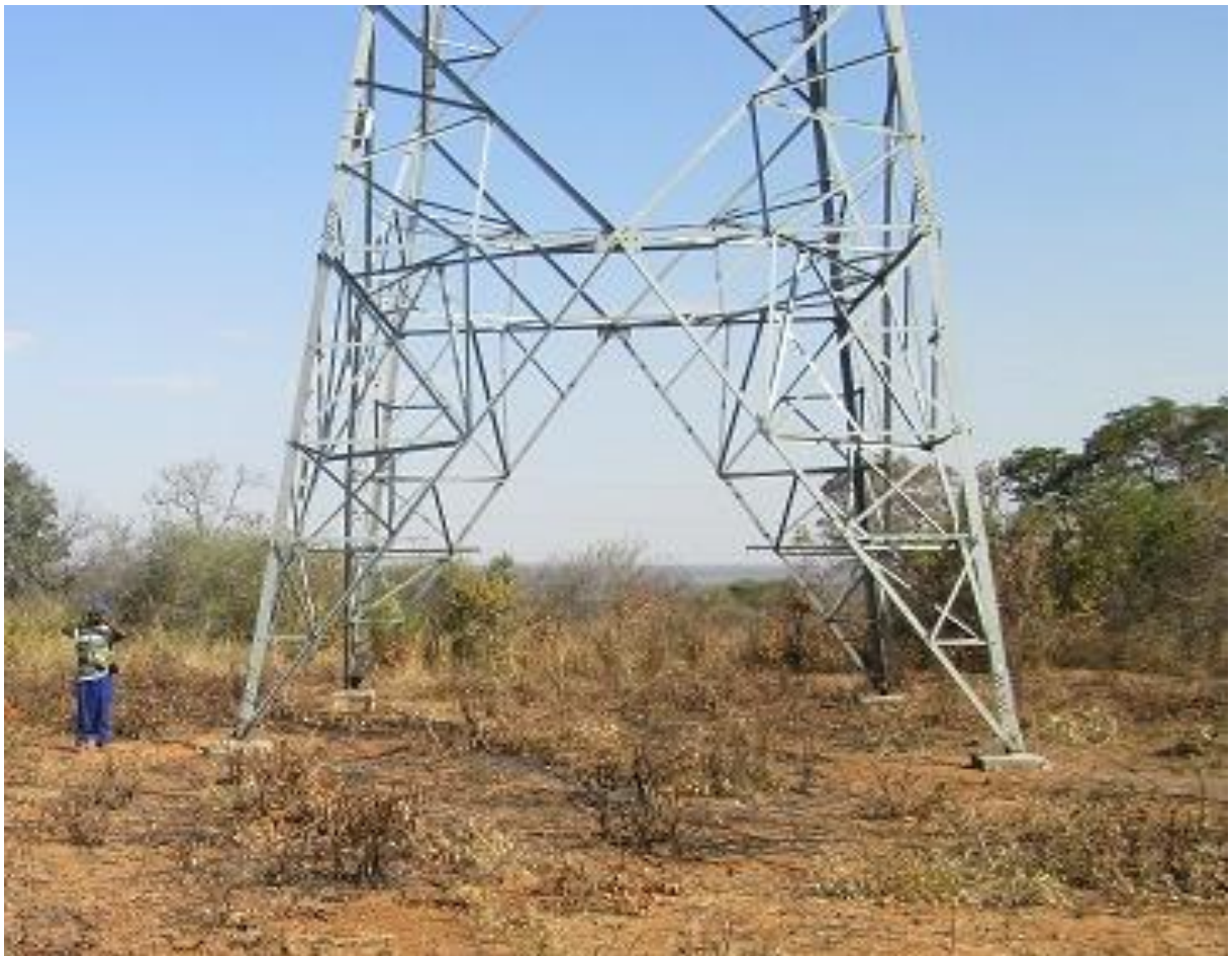
Figure 23: Self-supporting power transmission tower standing on four concrete foundation spots.
