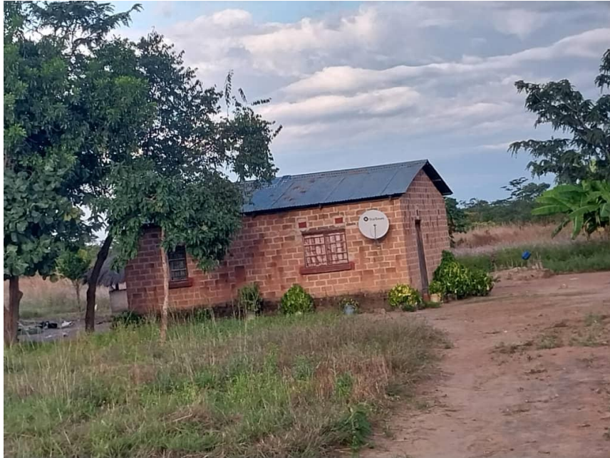
Plate showing Typical House in Community near the Project Area
