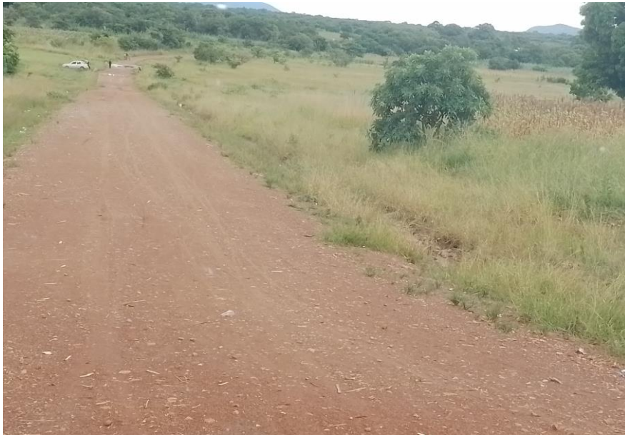
Plate showing Typical road used by communities near project area
