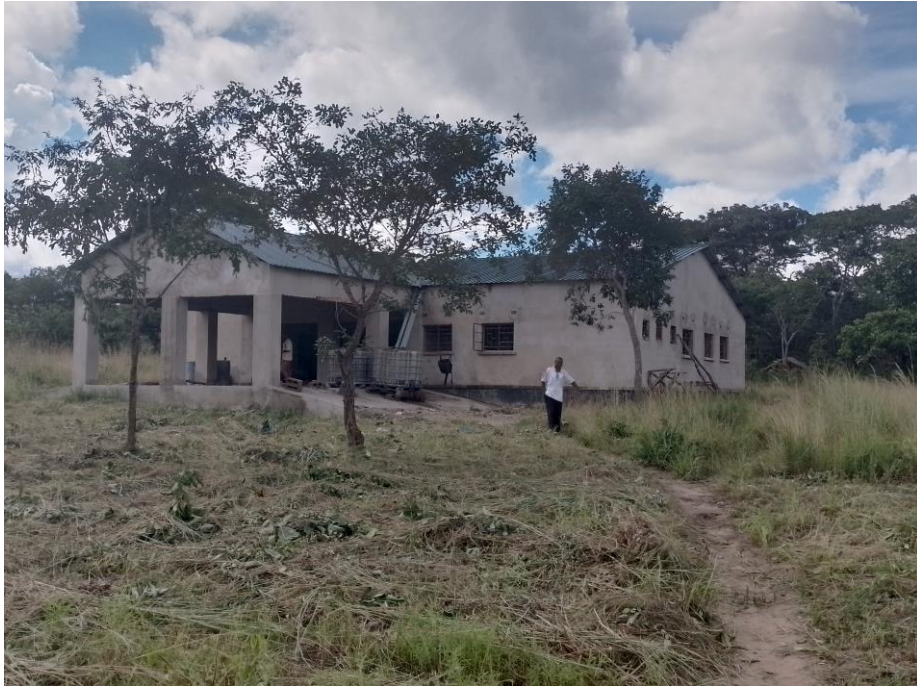
Plate showing the Health Post being constructed at Nazareth
