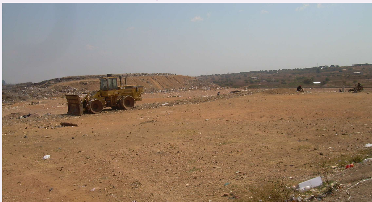
Chunga Landfill in Lusaka
